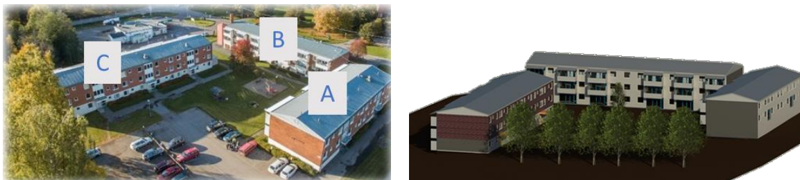
Figure 36. Three buildings in the cluster for renovation in Ludivika, Sweden
