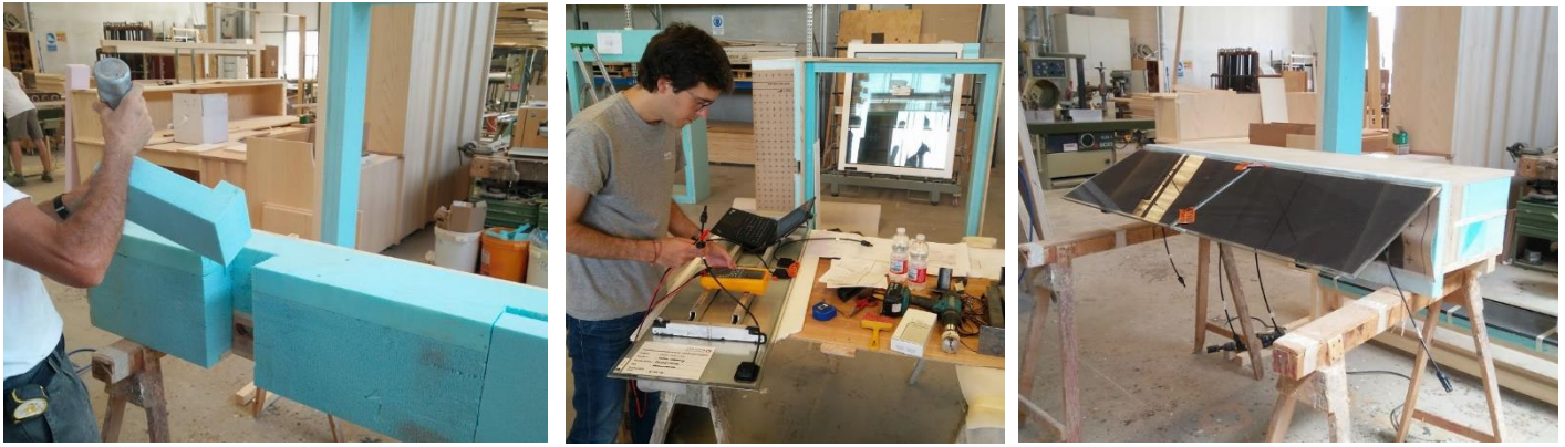
Figure 11. Manufacturing and checks of PV and air ducts (Source: Eurofinestra)
